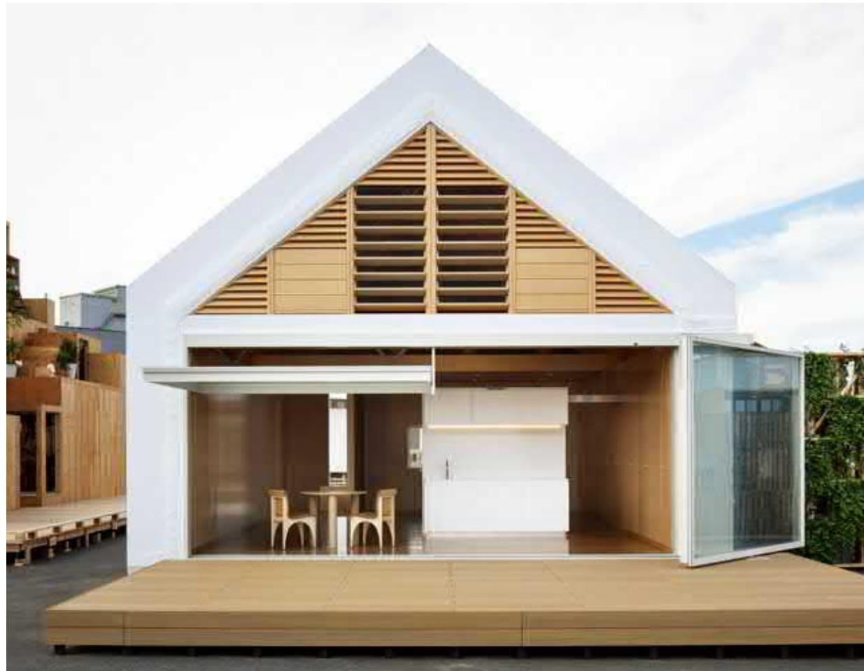
Mechanically louvred windows create the openness that gives Shigeru Ban's house its name.
