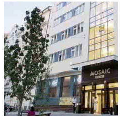
Hotels. Prague's Hotel Mosaic House is not only fitted out with various Hansgrohe products, but also runs the Pontos AquaCycle and Pontos HeatCycle.
